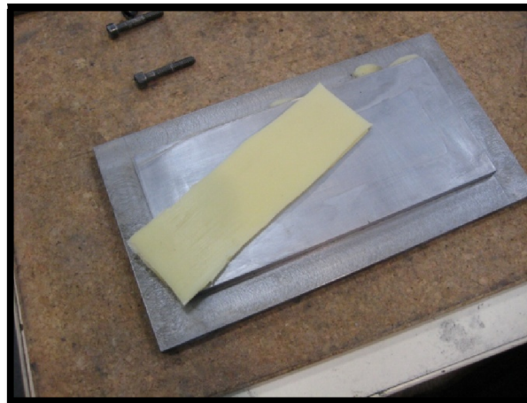
Figure E 17 – Completed adhesive plate removal.
