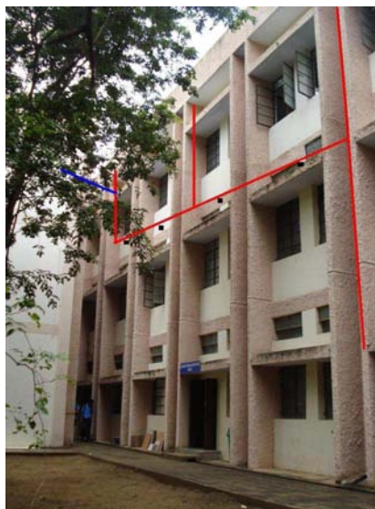
Picture 3 – Conveyance system
