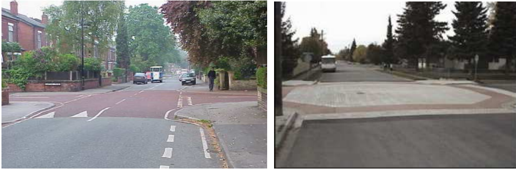
Fig.3.14 – Plataformas sobreelevadas (fonte: http://www.trafficcalming.org/centerislandnarrowrings.html )
