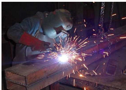
Fig. 4.17 – Soldadura MIG-MAG [38]
