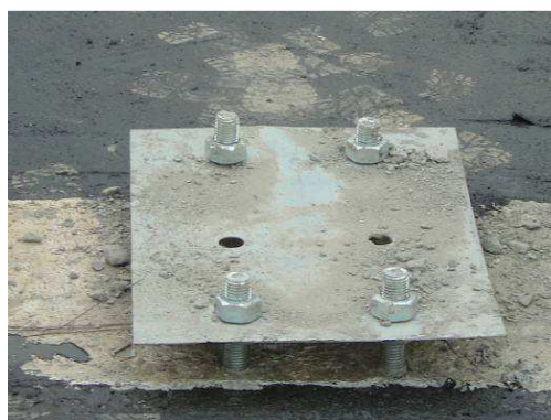
Fig. 6.17 – Pormenor dos chumbadouros
