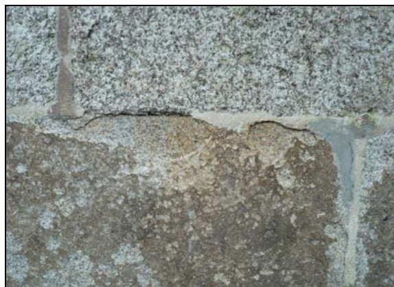
Quartel-General do Porto
