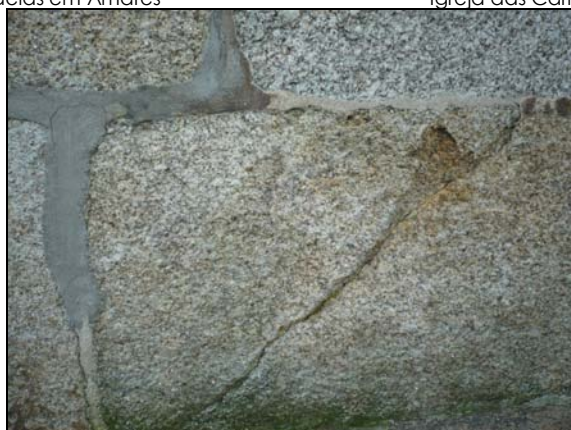
Quartel – General do Porto
