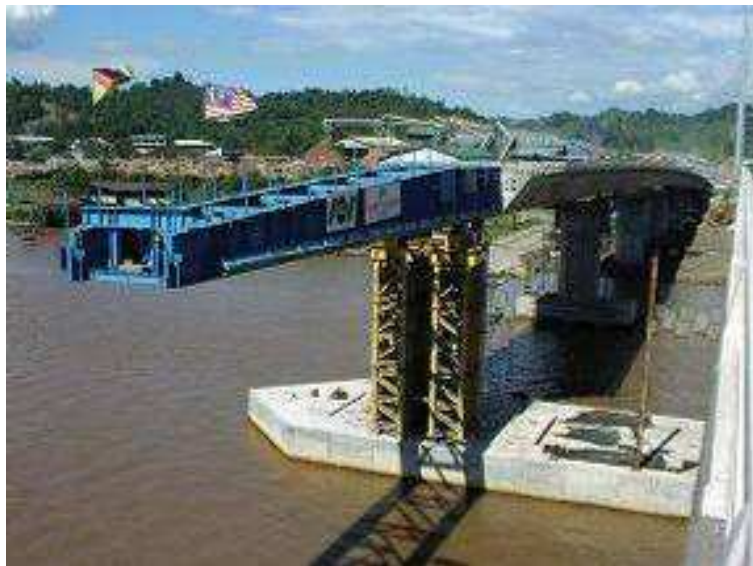
Fig. 2.24 – “Avant-bec” (Kemena Bridge Malaysia) [18]
