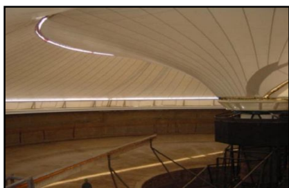
Fig.3.20. – Valenton Water Treatment Plant
