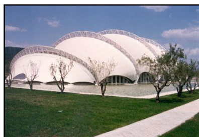
Fig.3.21. – Venafro Chemical Research Centre
