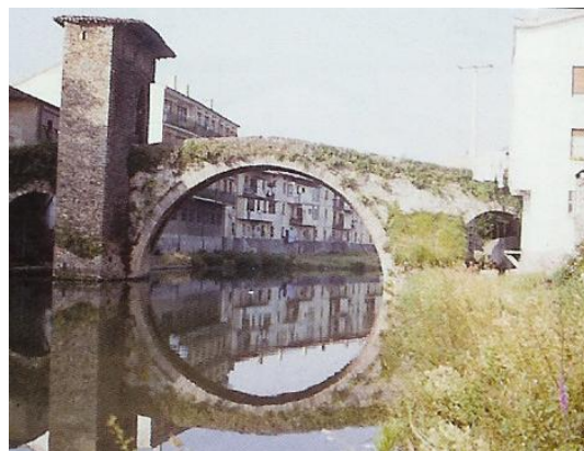
Fig. 2-27 – Ponte Valmaseda, arco de volta perfeita (Fernandez (2004))
