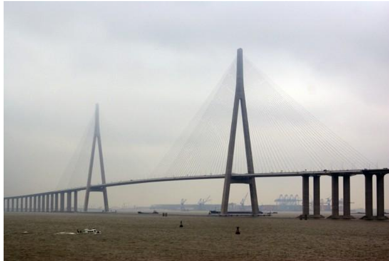
Figura 2.6 - Ponte Sutong, China (Janberg, 2009)
