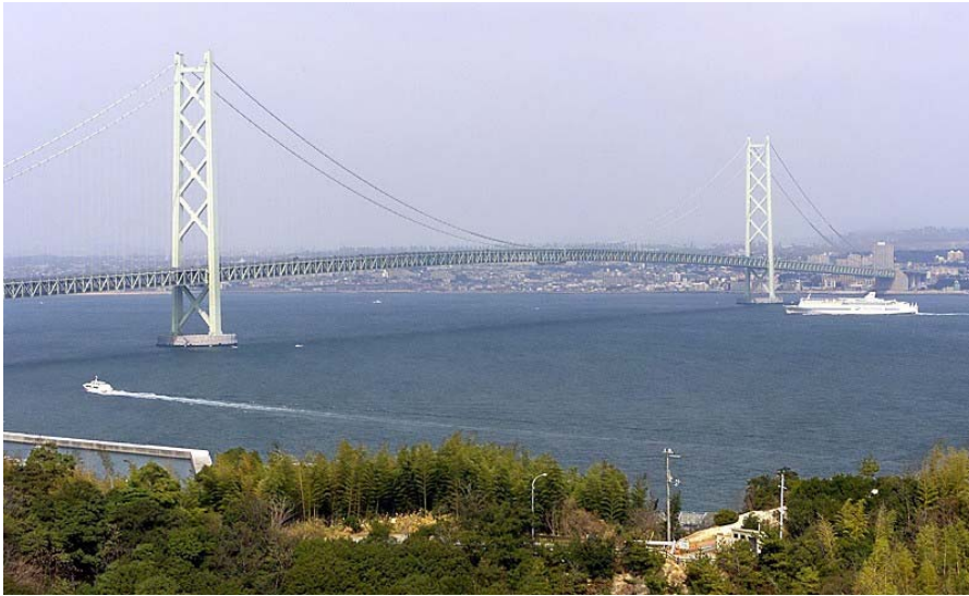
Fig. 2.3 Akashi-Kaikyo Bridge, Japan
