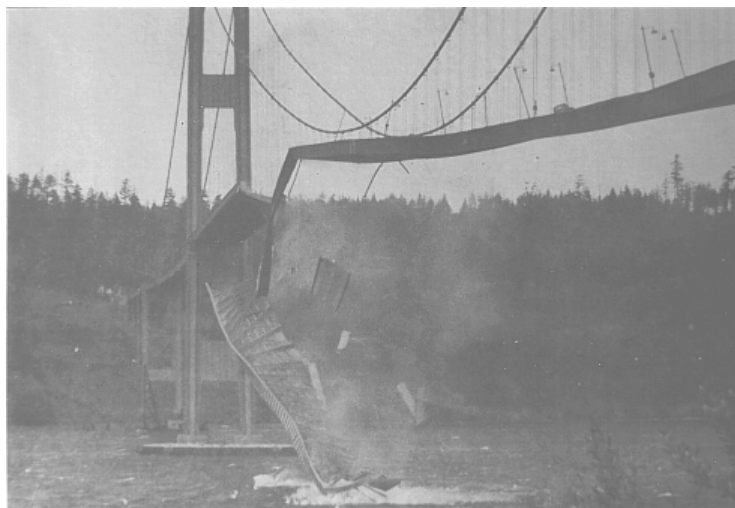
Fig. 2.2 Collapse of Tacoma Narrows Bridge
