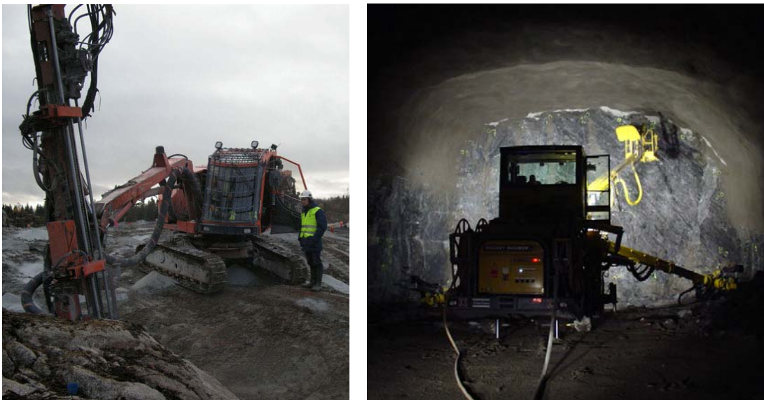
[fig73] – Surface and underground drilling tests
