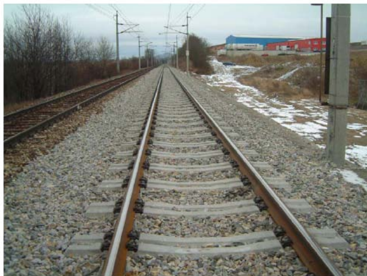
Fig 15 “Frame sleeper” Böheimkirchen (workshop track for high speed railways, 2006)
