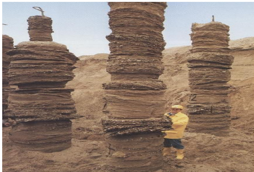
Fig 3.4 - Colunas de jet grout (Bilfinger Berger Foundations)
