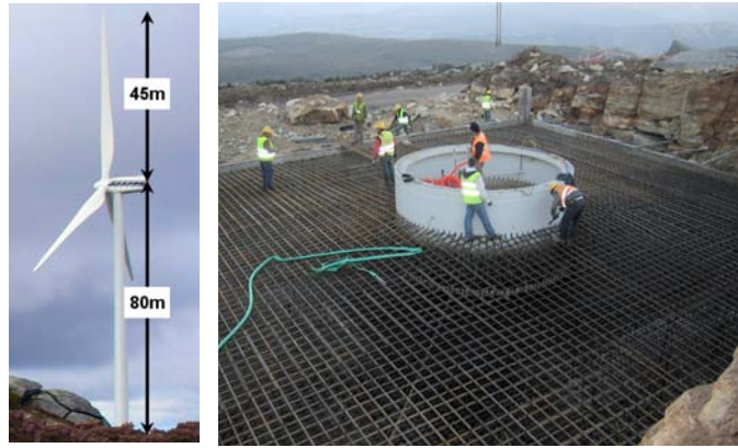
Figure 6.1: Wind tower and RC foundation
