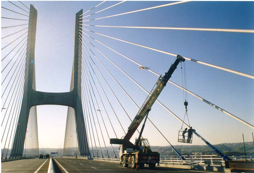
Fig. 6: Installation of accelerometers on stay cables
