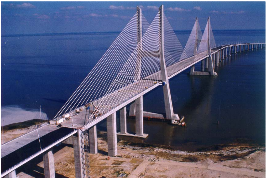
Fig. 2: Vasco da Gama cable-stayed bridge
