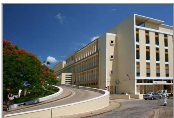
Figura 6: Hospital Central de Maputo
