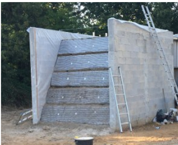
Fig. 1. Full-scale geosynthetic-reinforced slope (GRS) constructed under the CDW_LongTerm research project.
