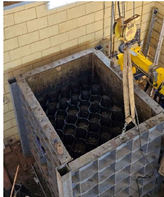
Fig. 4. View of the geocells inside the test box.
