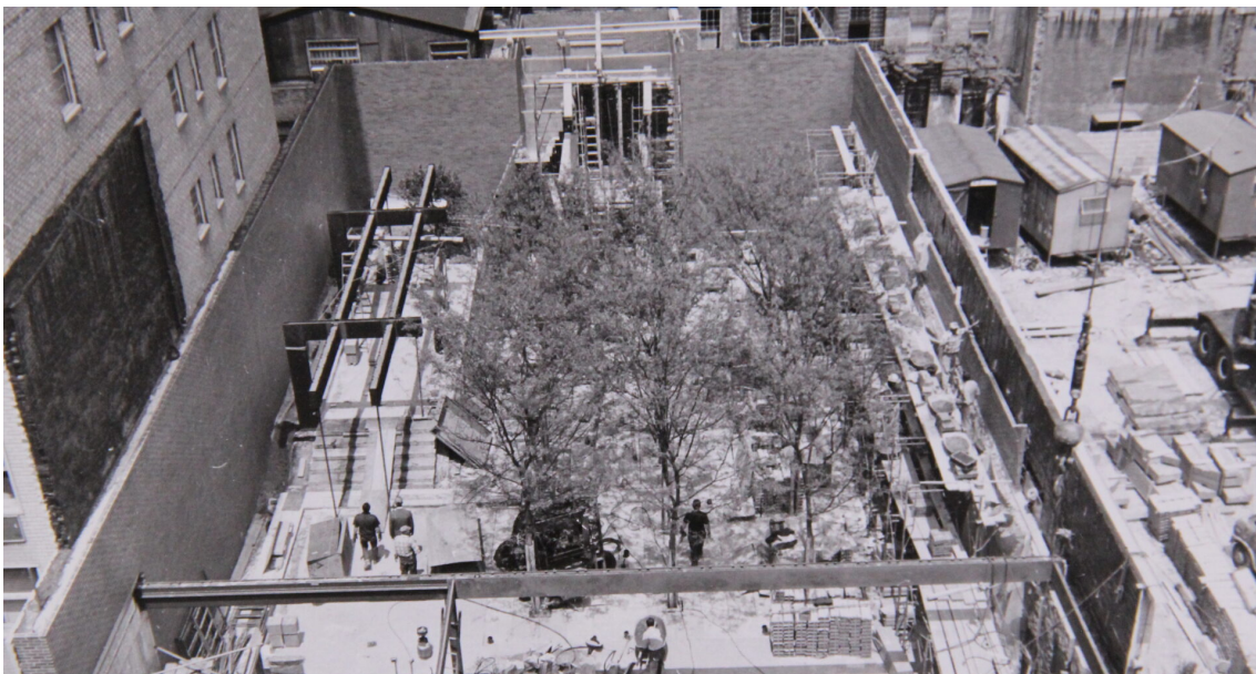
Figure 17 - Greenacre Park During Construction (1971) Source: Greenacre Foundation, n.d.
