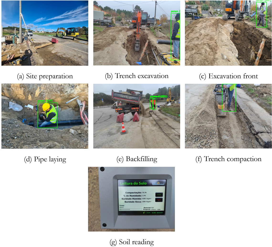
Figure 5.16: Examples of construction supervision images used in the AI image risk analysis workflow
