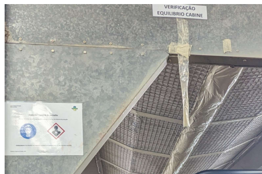
Figure 3.13: Qualitative visual indication of booth pressure balance using adhesive tape.
