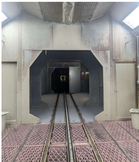
Figure 3.9: Painting booth: wet scrub
