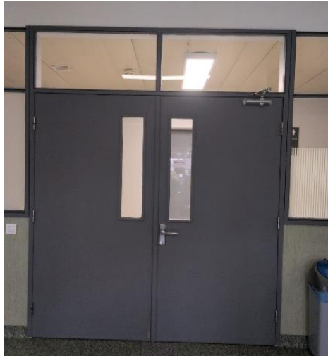
Figure 11: Open Bay – Exit Double Doors.
