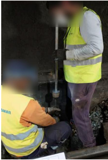
Figure 21 - LDP test in Juncal tunnel, execution project
