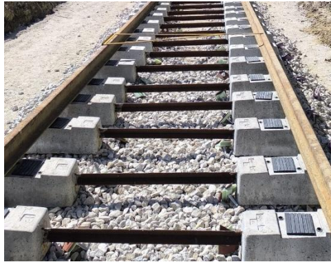
Figure 3 - Twin-block sleepers
