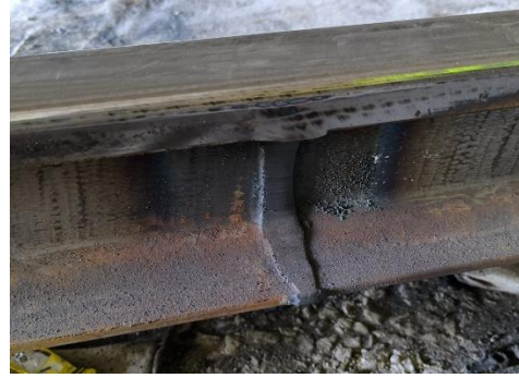
Figure 8 - Continuous welded rail
