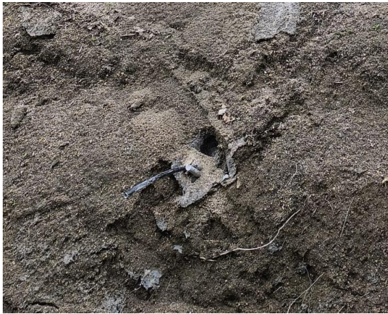
Figure 29 - Grouted soil nail
