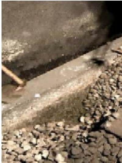
Figure 16 - Trial pit in the Juncal tunnel, preliminary campaign
