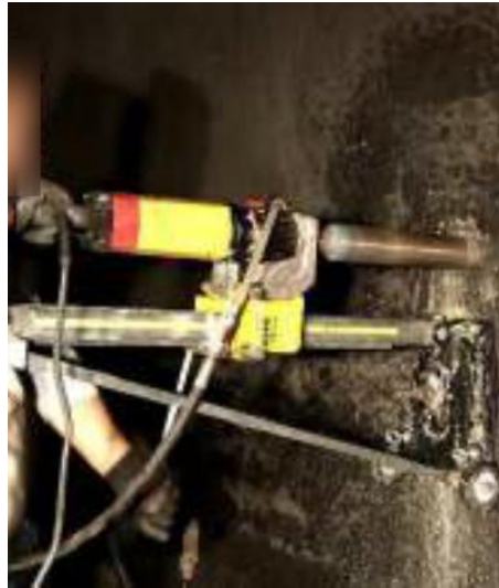
Figure 17 - Core drilling in the Juncal tunnel, preliminary campaign
