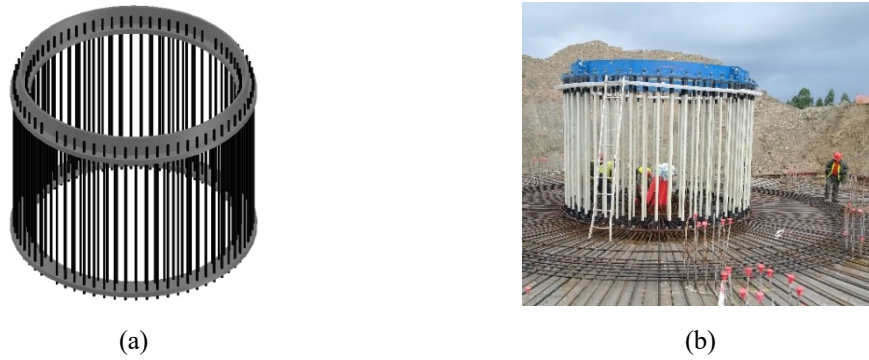
Figure 2.16 – Connection between steel tower and concrete foundation using the AC solution: (a) schematic drawing (b) onsite installation
