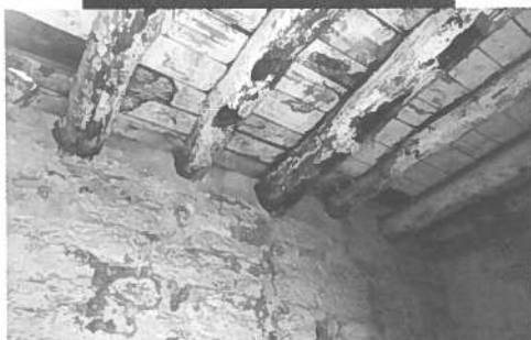
8. Whitewashed through-stone wall.
