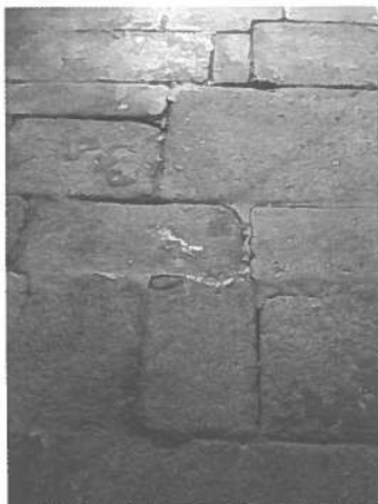
7. Granite paved wall.
