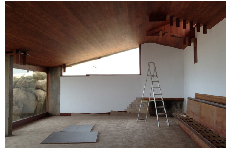
32. Conservation intervention on interior wood paneling.
