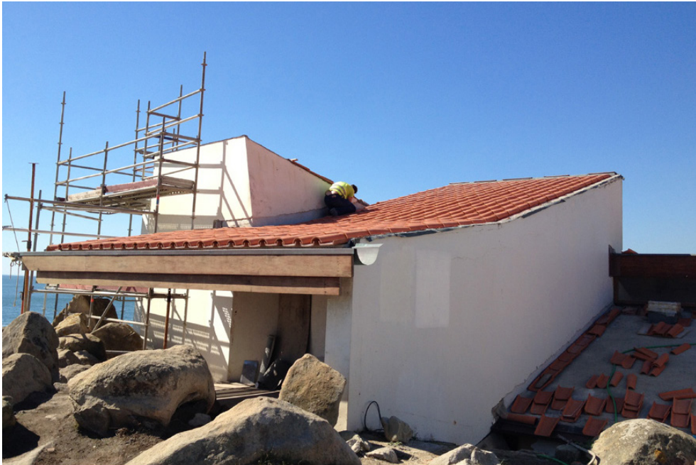
31. Replacement of the roof tiles.
