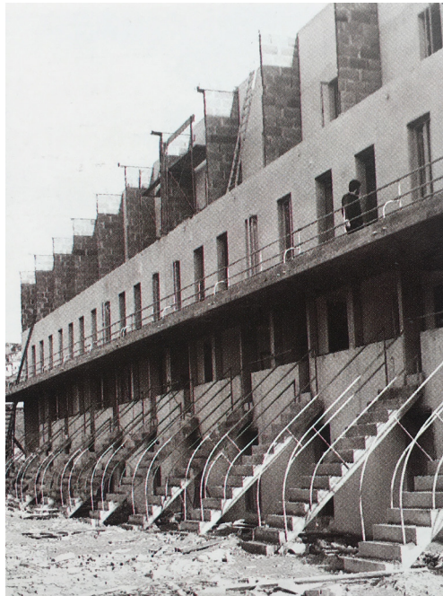
24. First phase of construction.
