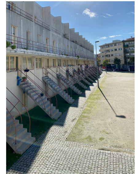
15. Individual staircases to access the dwellings..
