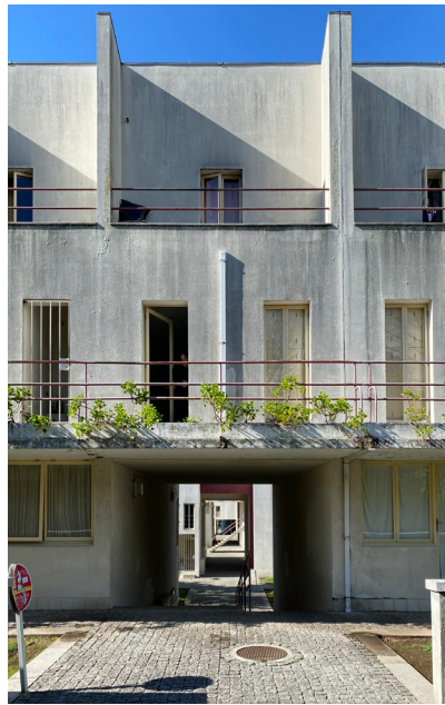
12. Passage through the housing blocks.
