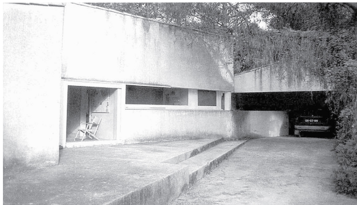
05. South façade and garage.
