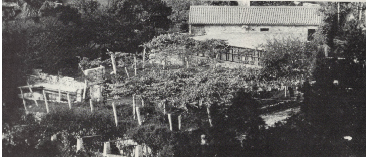
06. South façade and garden, 1979.
