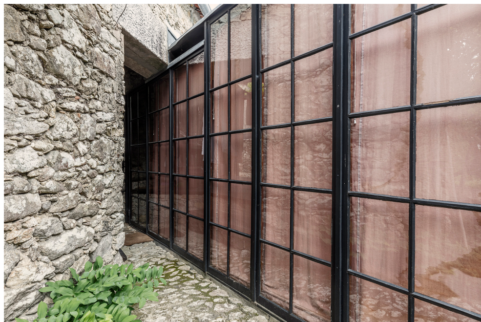
13. Contact between the curtain wall and the granite walls, 2023.
