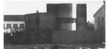
30. North façade during construction.
