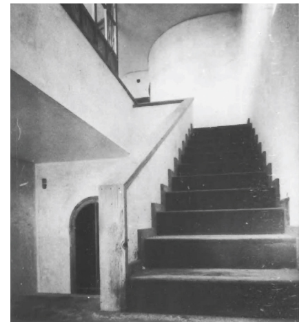
31. Interior staircase during construction.
