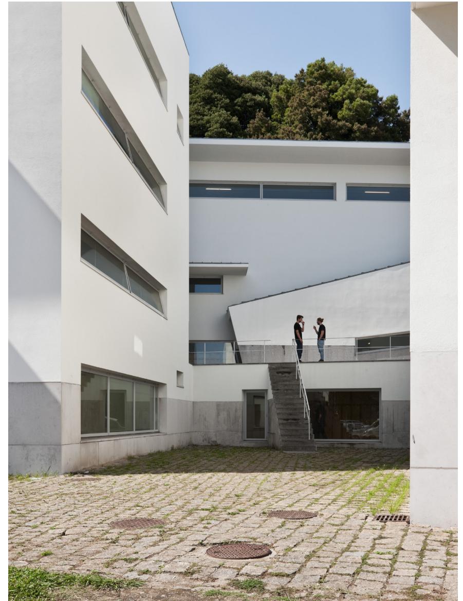
09. Main building entrance.
