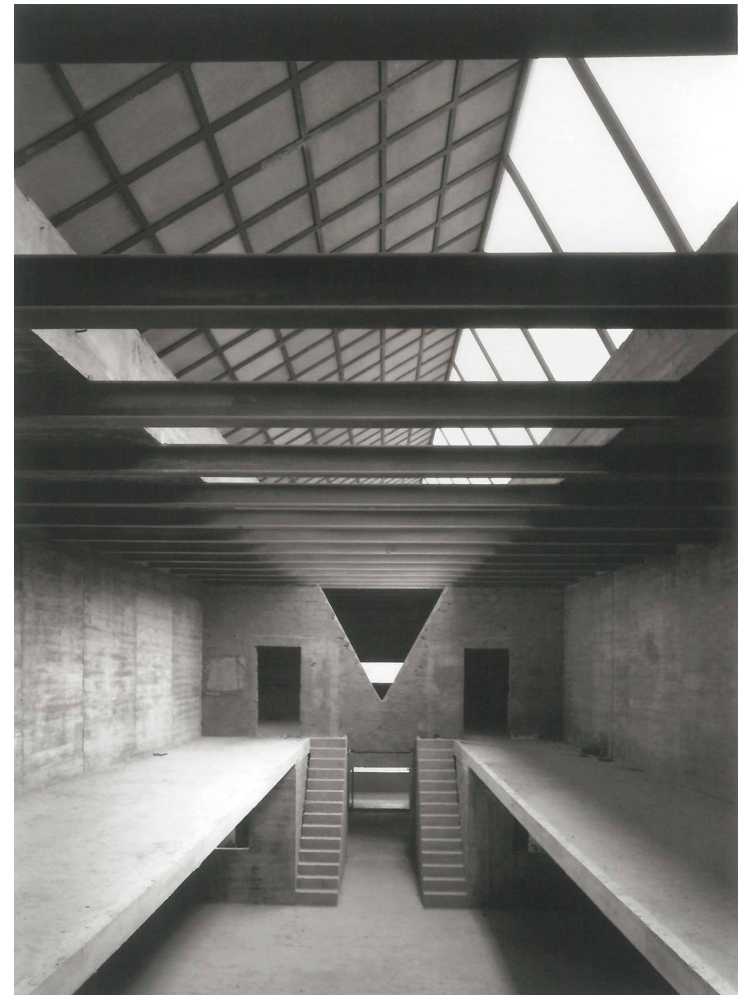
29. Library reading room during construction, 1993.
