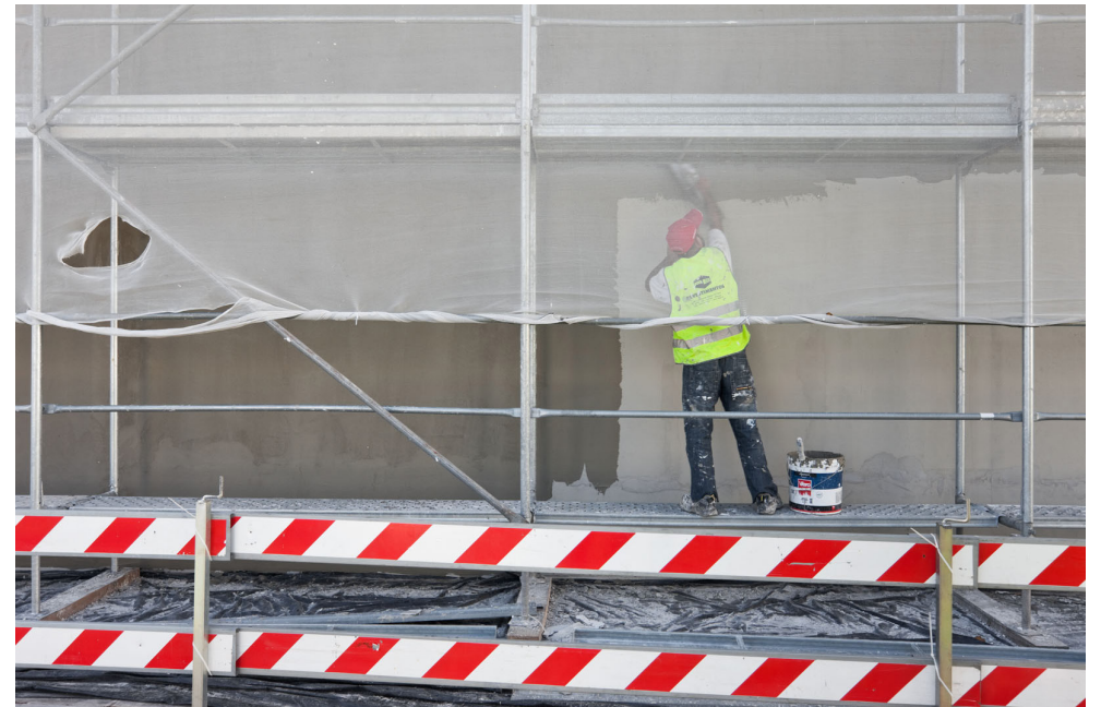
43. Replacement of the external coatings, 2016.
