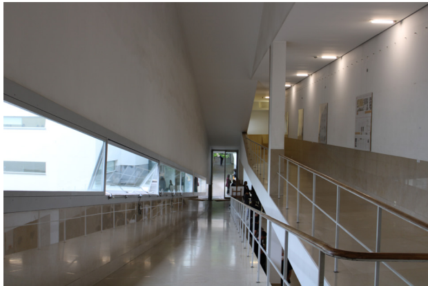
11. Main entrance ramp.
