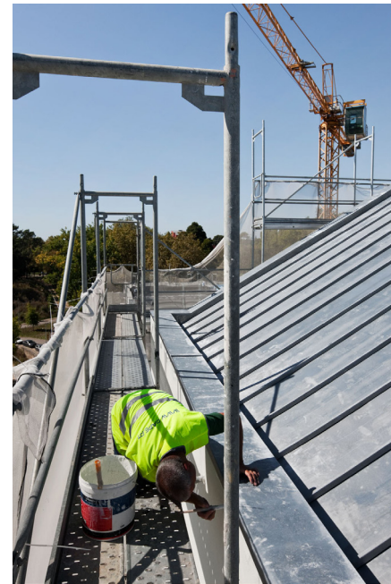
42. Intervention on the roofs, 2016.
