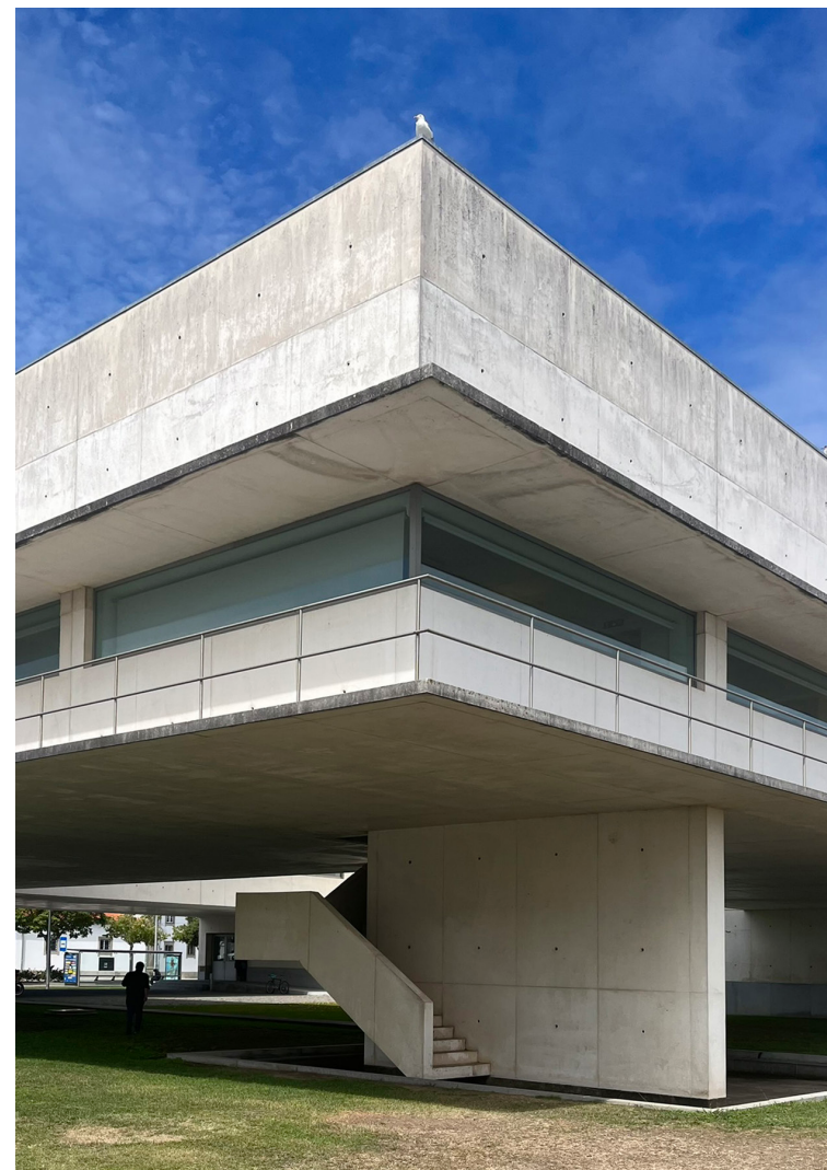
11. Southwest façade and staircase.
