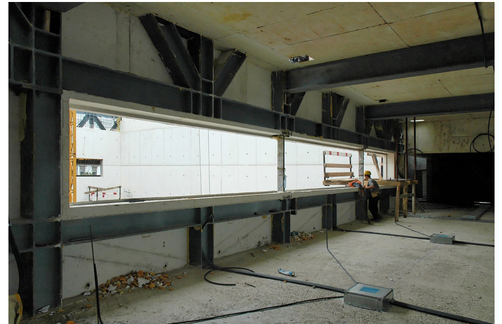
21. Interior during construction works.
