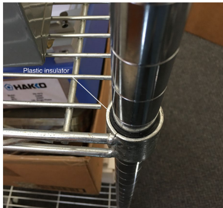
Figure 1.4: Example of unintended loss of grounding in storage infrastructure: plastic insulating rings at rack connector junctions can prevent proper grounding and allow electrostatic charge build-up during storage and handling. Extracted from: [4, p. 9]
