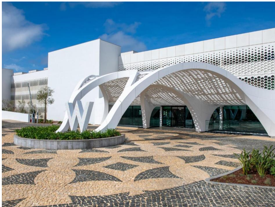
Figure 8. Photo of the complete porte-cochère of the W Algarve hotel featuring the robotically fabricated GRC components. Source: W Hotel Algarve
