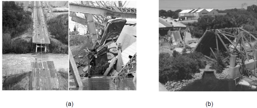
Figure 2.1: a) Collapse of the Silver Bridge, 1967. USA. b) Collapsed north section of the Minneapolis I-35W Bridge, Minnesota, USA. Adapted from (Figueiredo et al., 2011).
