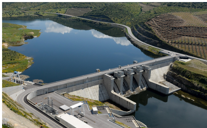
Figure 5.7: Overall view of the Feiticeiro dam.
