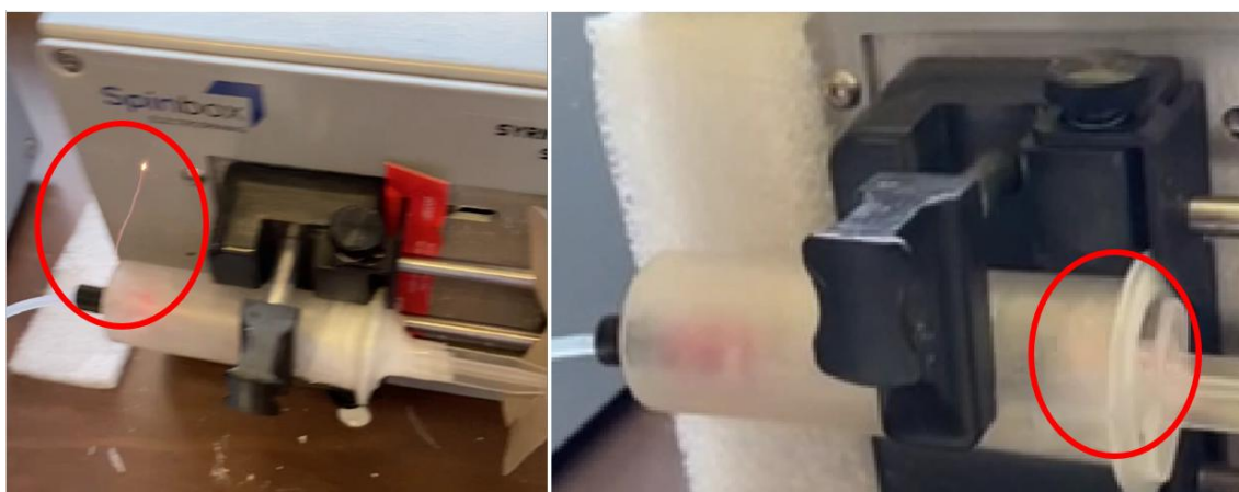
Figure 11 - Examples of arcing.
