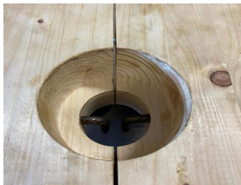
Fig. 23 - Downward-bent rebar + timber block.
