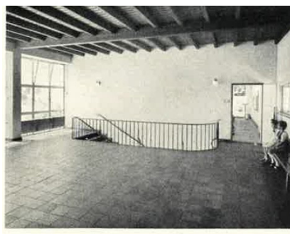
Recreation hall on first floor / Pausenhalle im I. Stock
