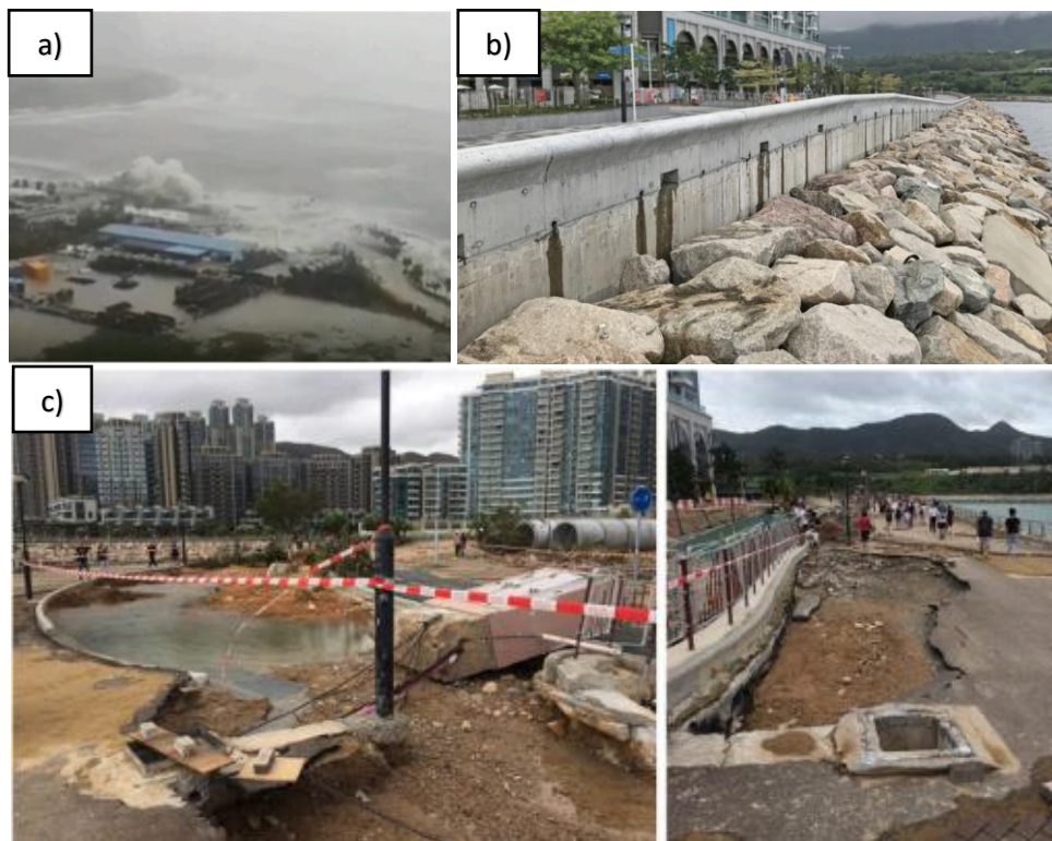
Figure 2.18 - Photos of the Tseung Kwan O waterfront park: (top left) wave overtopping during Mangkhut (video snapshot: https://www.youtube.com/watch?v=fmViQCDc1FM ); (bottom) damage to the promenade and waterfront facilities; (top right) wave wall built after Typhoon Mangkhut (modified from: https://www.devb.gov.hk/filemanager/en/content_1044/20200607_04.html ). (Qiang et al. , 2021).
