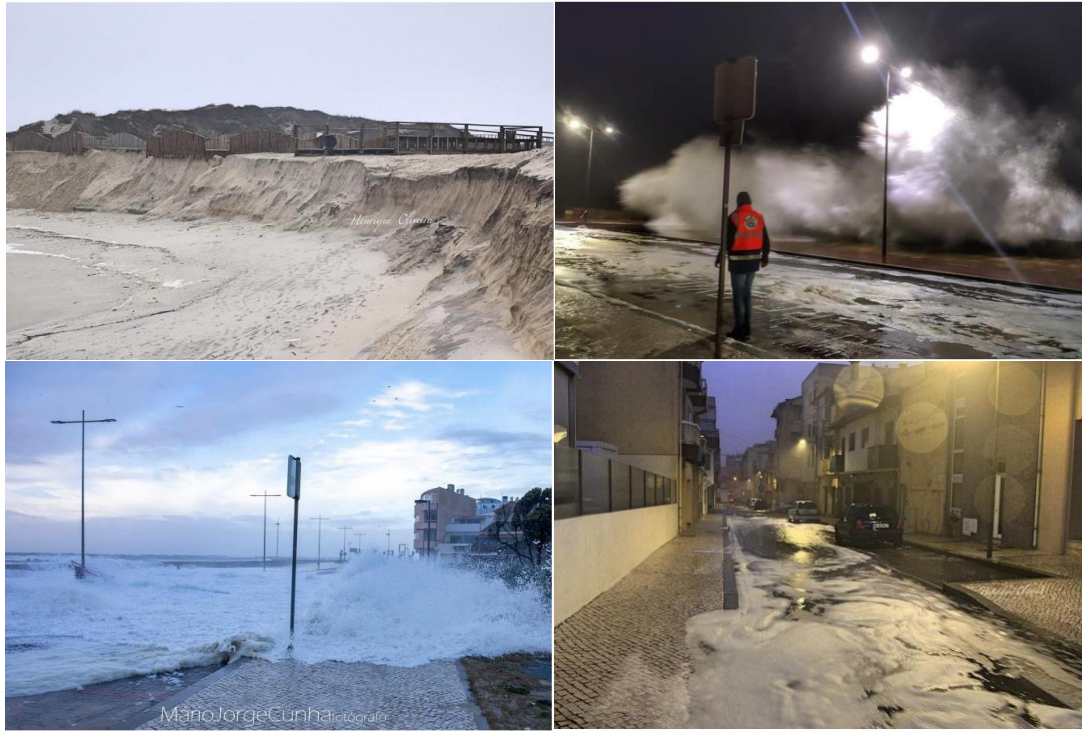
Figure 3.6 - Erosion of dunes, overtopping into the streets, saltwater in the streets and flooding (Câmara Municipal de Ovar, 2021).
