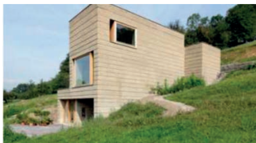
Figura 11 Austria – Schlins, Boltshauser Architekten, Martin Rauch, Rauch residential house, 2008 (foto di Beat Bühler)
