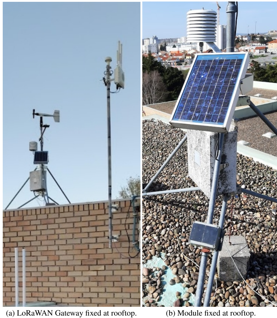
Figure 3.27: Fixation of the module outdoors close to the Gateway.
