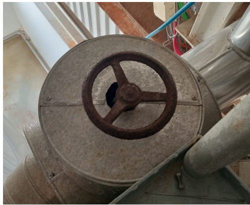
Figure 3.7: Control Valve (Manual actuation)
