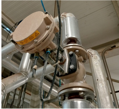
Figure 3.8: Control Valve (Diaphragm Actuation)
