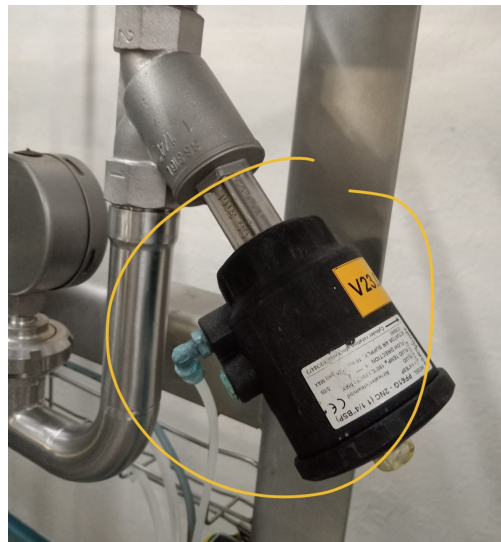
Figure 3.12: Angle Valve (Piston Actuation)
