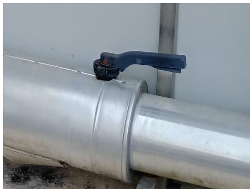
Figure 3.10: Butterfly Valve (Manual Actuation)
