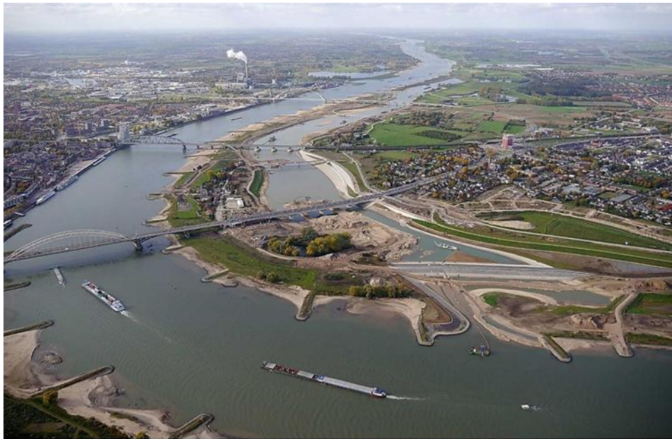
Fig. 19 - Aerial picture taken in 2016 after the completion of Room for the River plan in Nijmegen [54].
