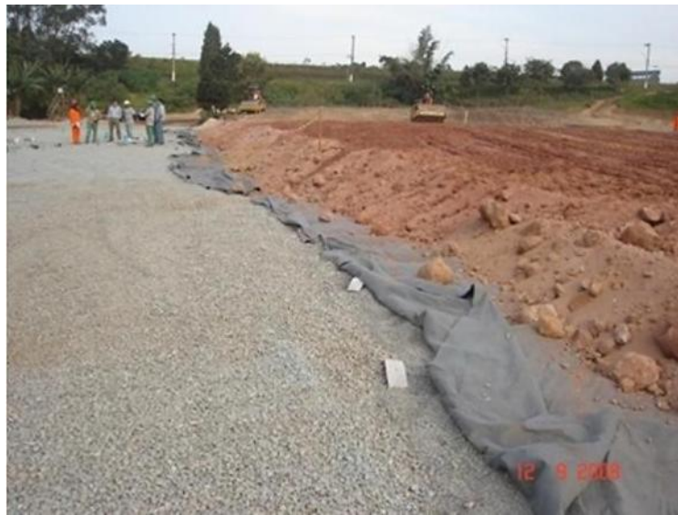
Fig. 14 - Installation of Bidim geotextile served as a separation layer between the drainage mattress and the backfill to be applied [46].
