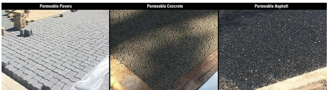
Fig. 12 - Three permeable pavement studied by USGS [41].
