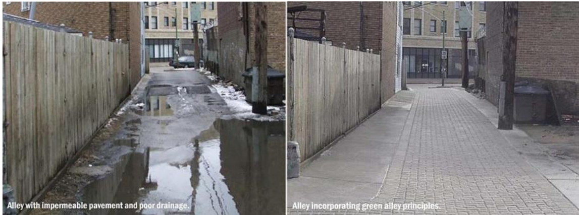
Fig. 11 - Road before and after alley incorporation was applied to a street in Chicago [39].
