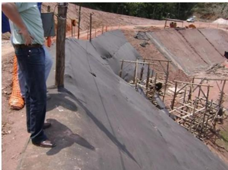
Fig. 15 - Bidim geotextile installation on slopes prior concrete coating [45].
