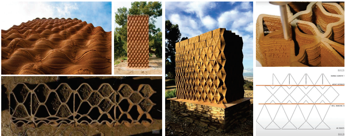
Figure 16 - The undulations of exterior wall surfaces can positively impact thermal performance. Left: Digital Adobe [84], right: TerraPerforma [85].
