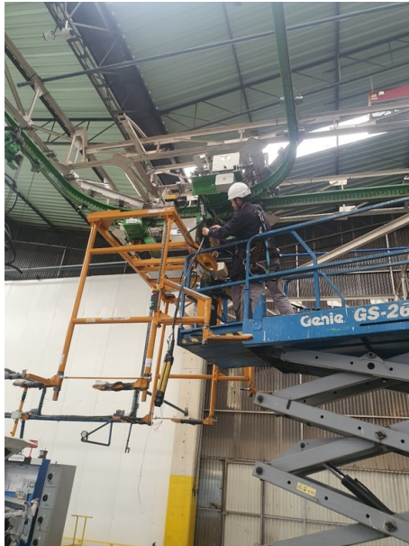
Figure C.18: Balancer System installation
