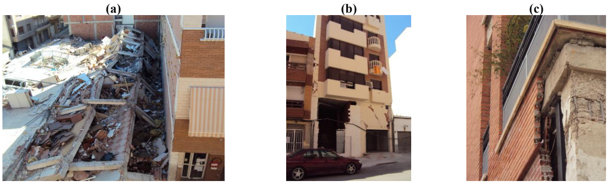
Figure 2-3: Lorca, Spain—2011: (a) building collapse after the earthquake; (b) building with a soft-storey mechanism; (c) column failure due to inadequate detailing of the transverse reinforcement
