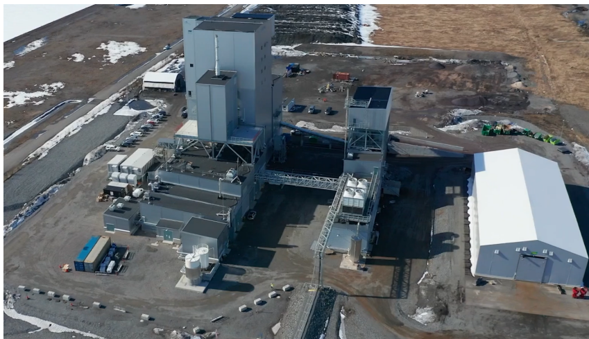
Figure 3.1: Hydrogen Storage Plant in Svartöberget, Luleå, Sweden [29]
