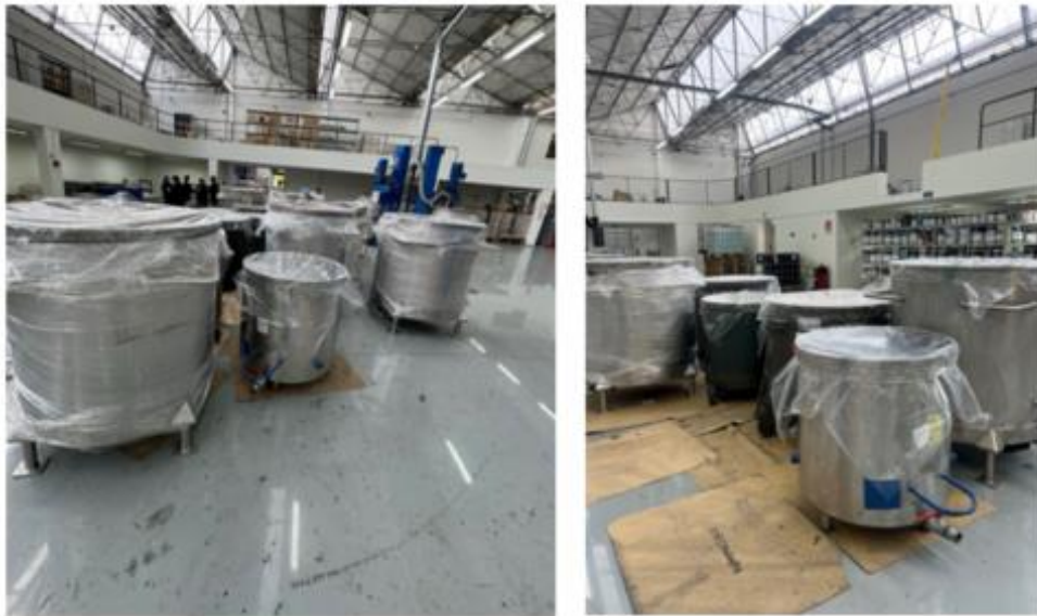
Figure 13 – Current situation in mobile tank storage area
