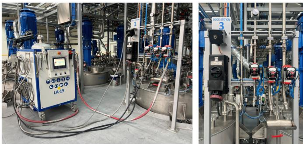
Figure 21 – Connection to Dock Station
