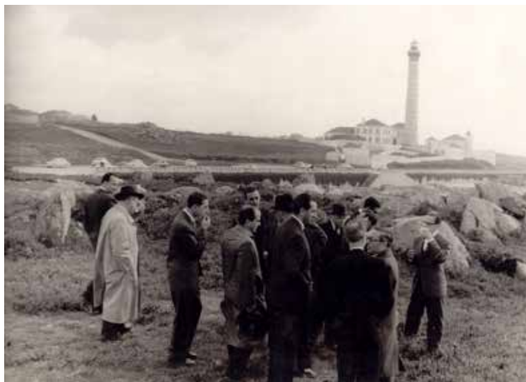
8. Fernando Távora and Alvaro Siza visiting the site where the Casa de Chã would be built in Boa Nova in the late 1950s (FIMS/AFT).
