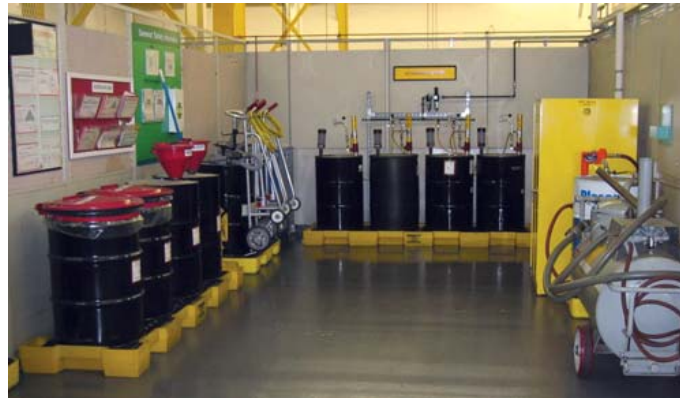
Figure 2.4: Lubricant Storage Room (Machinery Lubrication, n.d.)
